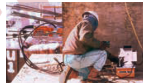
The PE60 used for pre-stressing.
