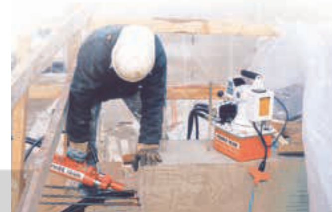
The PE60 used for pre-stressing.
